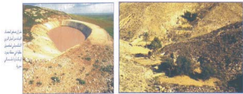
Fig. 7: Rainfall harvesting system at the topographic depressions
