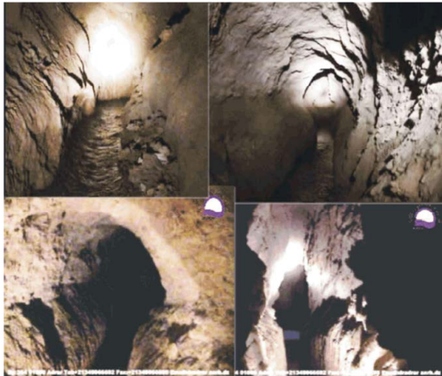
Fig. 10: The underground channel
